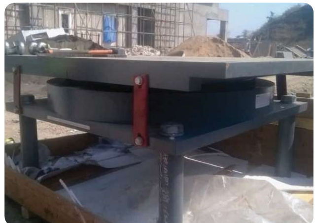
POT PTFE BEARING WITH 3000 TONS CAPACITY FOR NAGPUR CANCER HOSPITAL
