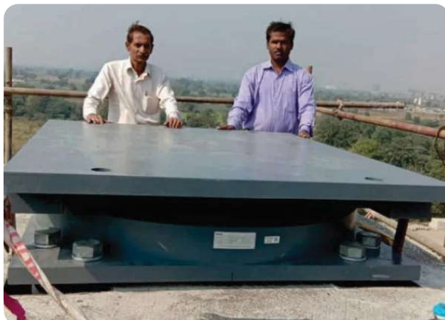
POT PTFE BEARING WITH 3000 TONS CAPACITY FOR NAGPUR CANCER HOSPITAL
